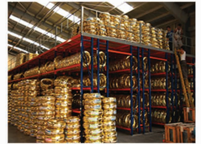
RACK SUPPORTED MEZZANINE
